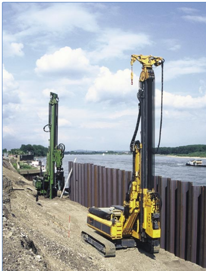
Driving steel sheet pile displaces soil with minimal excavation requirements.
