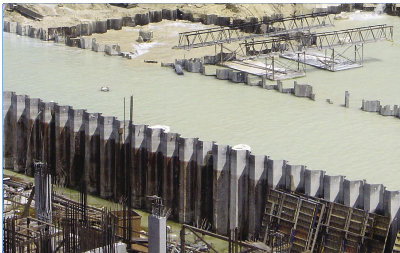
Steel sheet piling form continuous walls that are earth-tight and water resistant.
