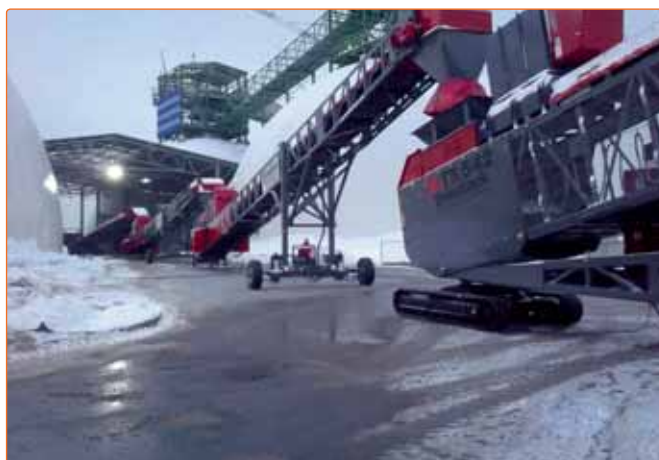
Mobile hopper feeder and link conveyors feeding ship loader
